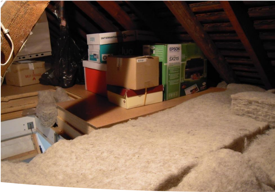
Between and above rafters. Rigid storage platforms.
