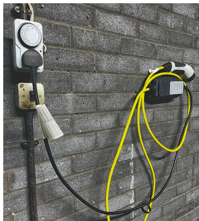
Garage charge point. Note the domestic 13 amp plug (Photo: Ivan Berg)
